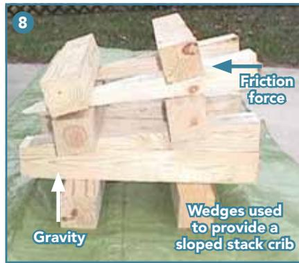
ratio). For example, if the footprint of modified stack cribbing is 12 inches, the safe height of the column is limited to 12 inches. Stack cribbing should form columns that support the load. The pieces should be aligned vertically to form such a column and provide the required strength.
